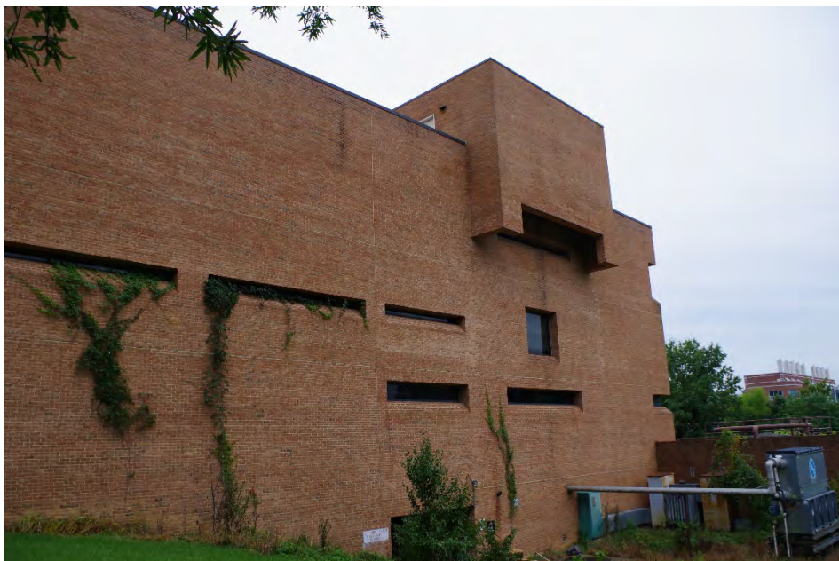
Photo 14 of 47: Northwest Façade, camera facing south.
