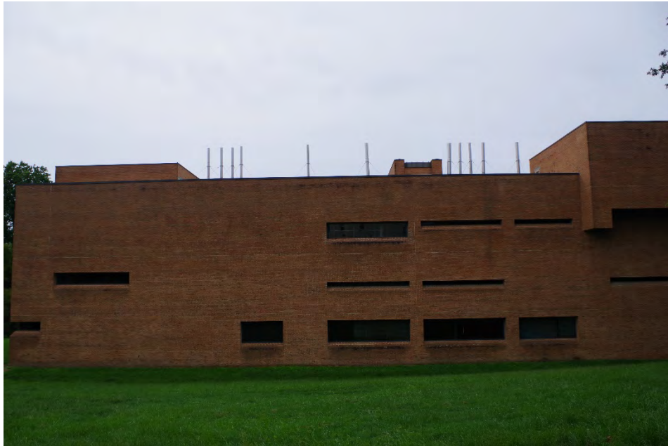
Photo 19 of 47: Overview of Northeast Façade, camera facing south-southeast.
