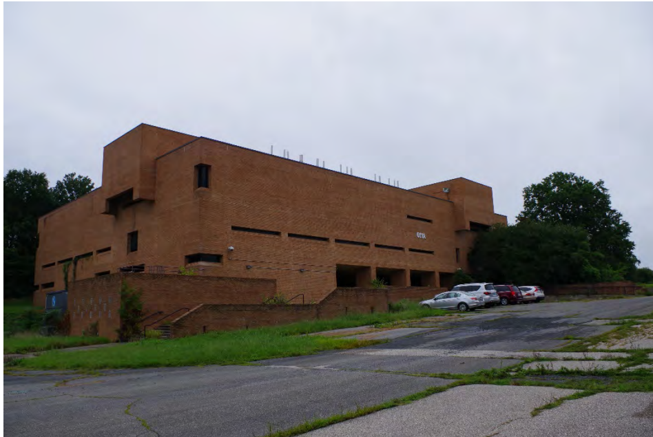
Photo 7 of 47: Overview of PG: 61-87, camera facing northeast.
