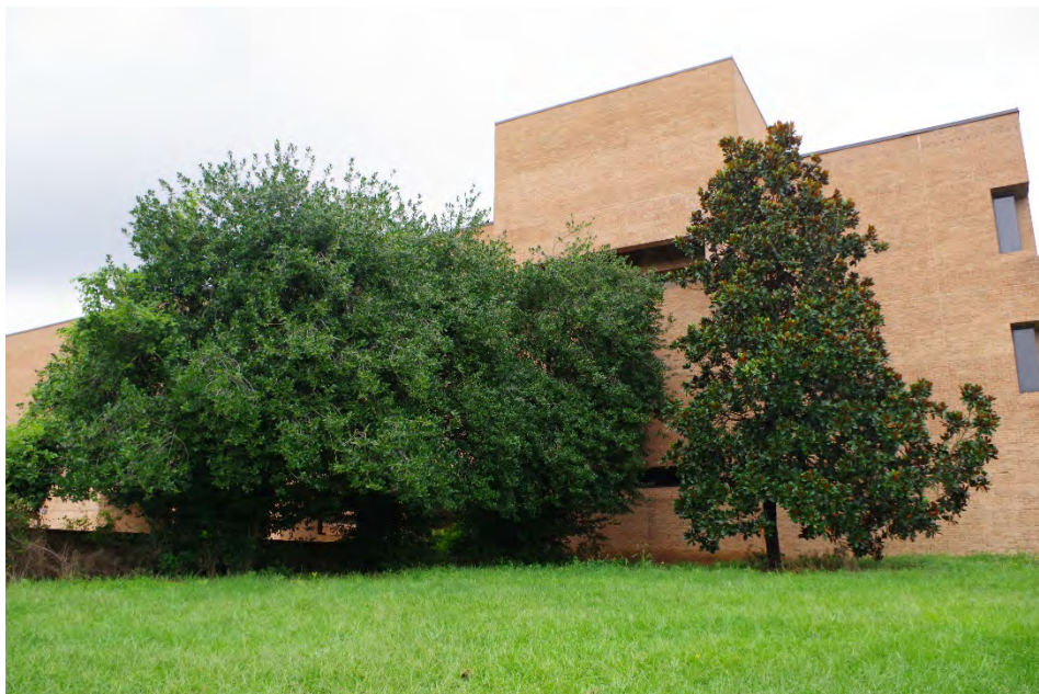
Photo 2 of 47: Oblique Overview, camera facing north.
