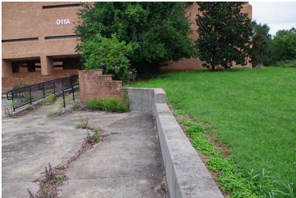
Photo 4 of 47: Overview of Entrance, camera facing north.
