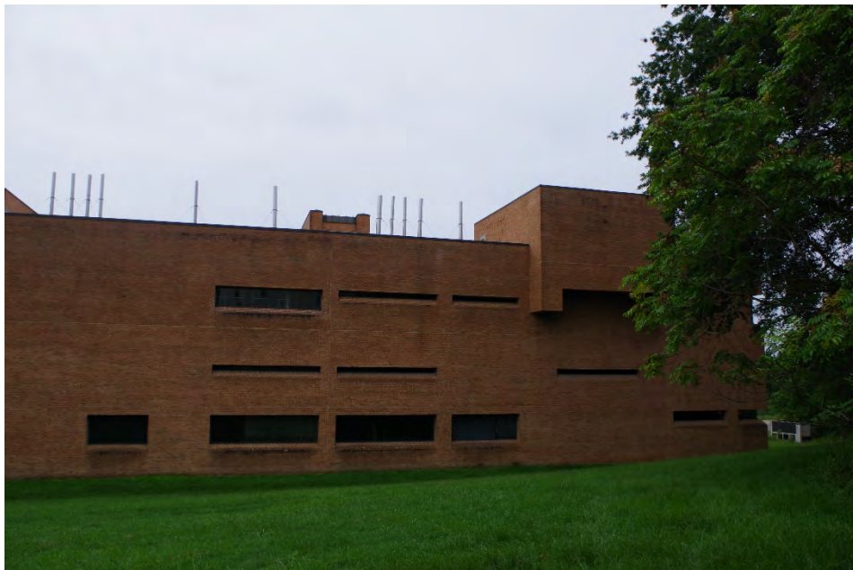
Photo 20 of 47: Overview of Northeast Façade, camera facing southeast.
