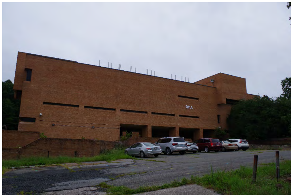
Photo 6 of 47: Overview of PG: 61-87, camera facing northeast.
