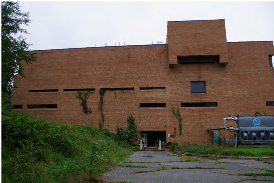
Photo 12 of 47: Lateral Overview of Northwest Façade, camera facing east-southeast.
