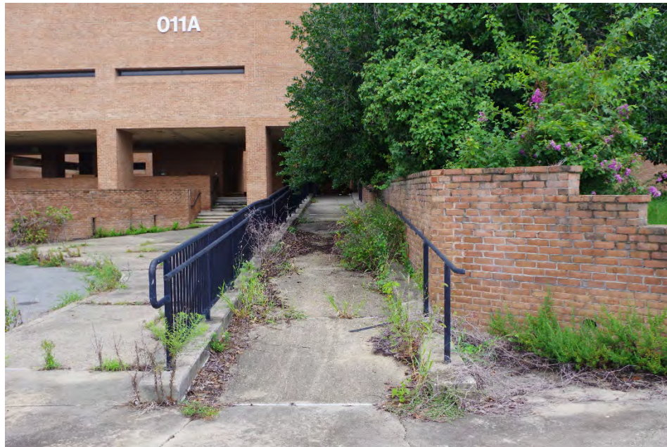
Photo 5 of 47: Overview of Entrance, camera facing north.
