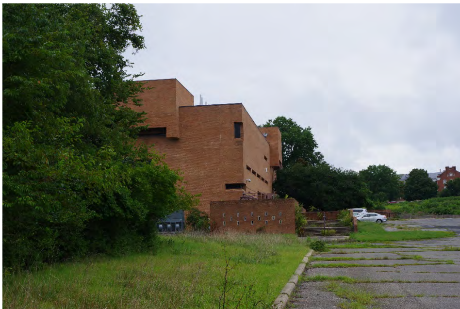
Photo 10 of 47: Overview of PG: 61-87, camera facing northeast.
