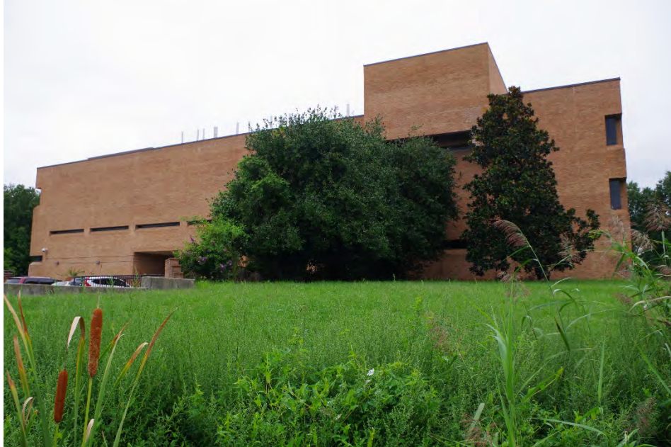
Photo 1 of 47: Front Façade, camera facing north.
