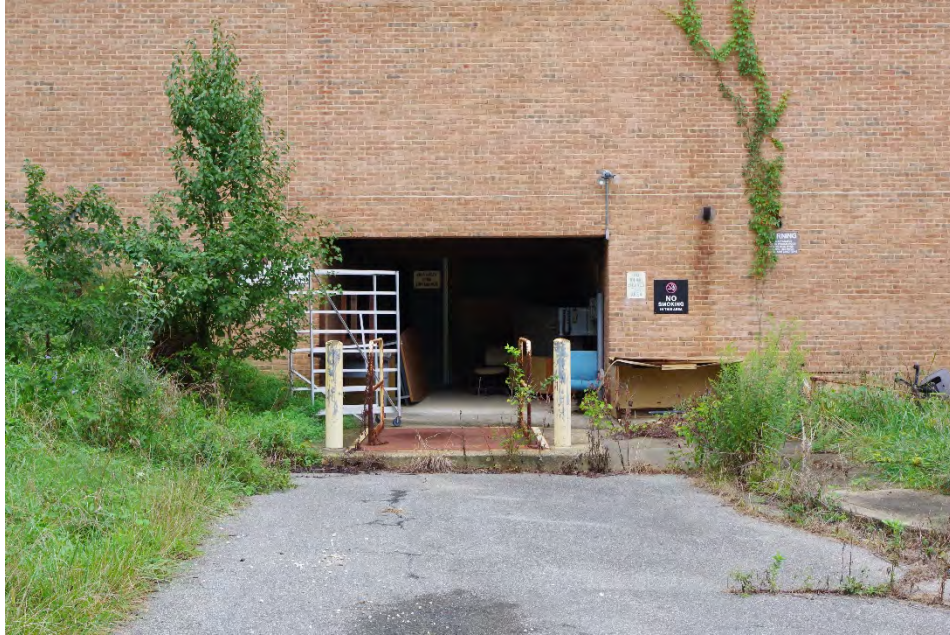
Photo 15 of 47: Entry on Northwestern Façade, camera facing southeast.
